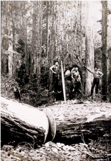
Lumbering spruce, falling, bucking or sawing apart, rounding edge, Mason Co., Washington. Image courtesy of Collier, Yale University Lantern Slide Collection.
