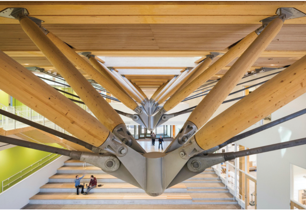
John W. Olver Design Building at the University of Massachusetts, Amherst. Photo courtesy of Albert Vecerka/Esto.
