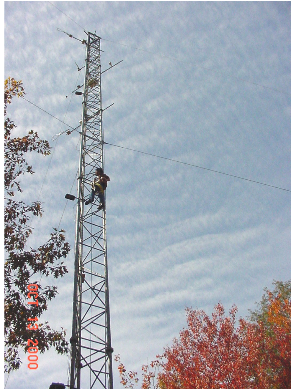
Researcher climbing the tower to adjust equipment. In order to operate properly, all instruments must be positioned well above the surrounding tree canopy line, yet within range of the average wind speed for the area, so as to collect data consistent with other flux towers.
