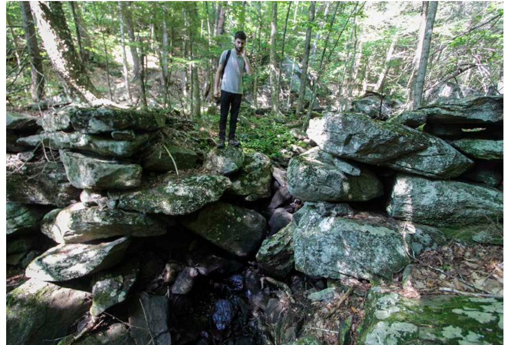
Dam site for the millpond at the Brown Brook sawmill. The stones are impressive in size and number. The site was built on a massive investment in human labor.
