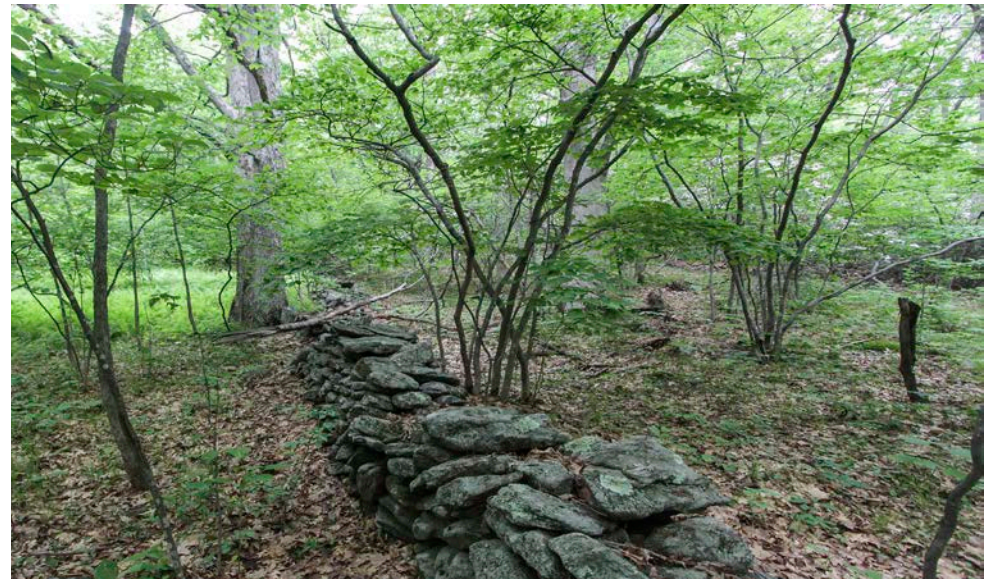
Well-preserved stone fence along the northeast border of the Dorman site illustrates the quality of work that went into fence construction. On top of this would have been wood or other material to attain the height necessary for keeping animals penned. 41°56'29.14"N; 73°15'57.90"W
